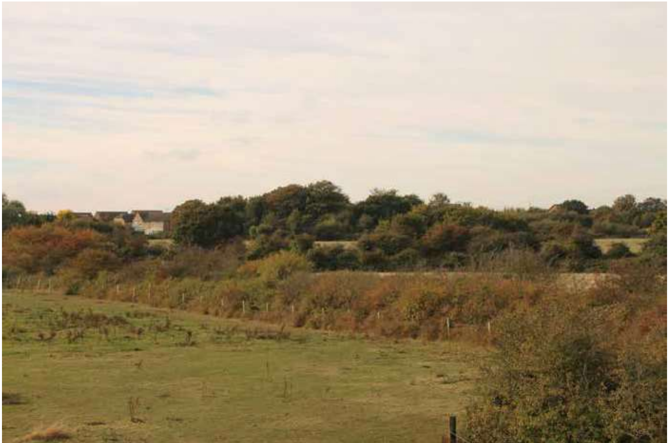
View 3: View of the battery from the east on the seawall, showing the tree and shrub growth on the scheduled monument.
