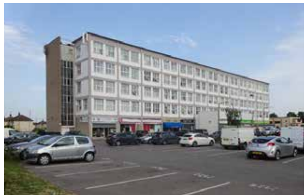
Figure 30: Car Park at Stamford House
