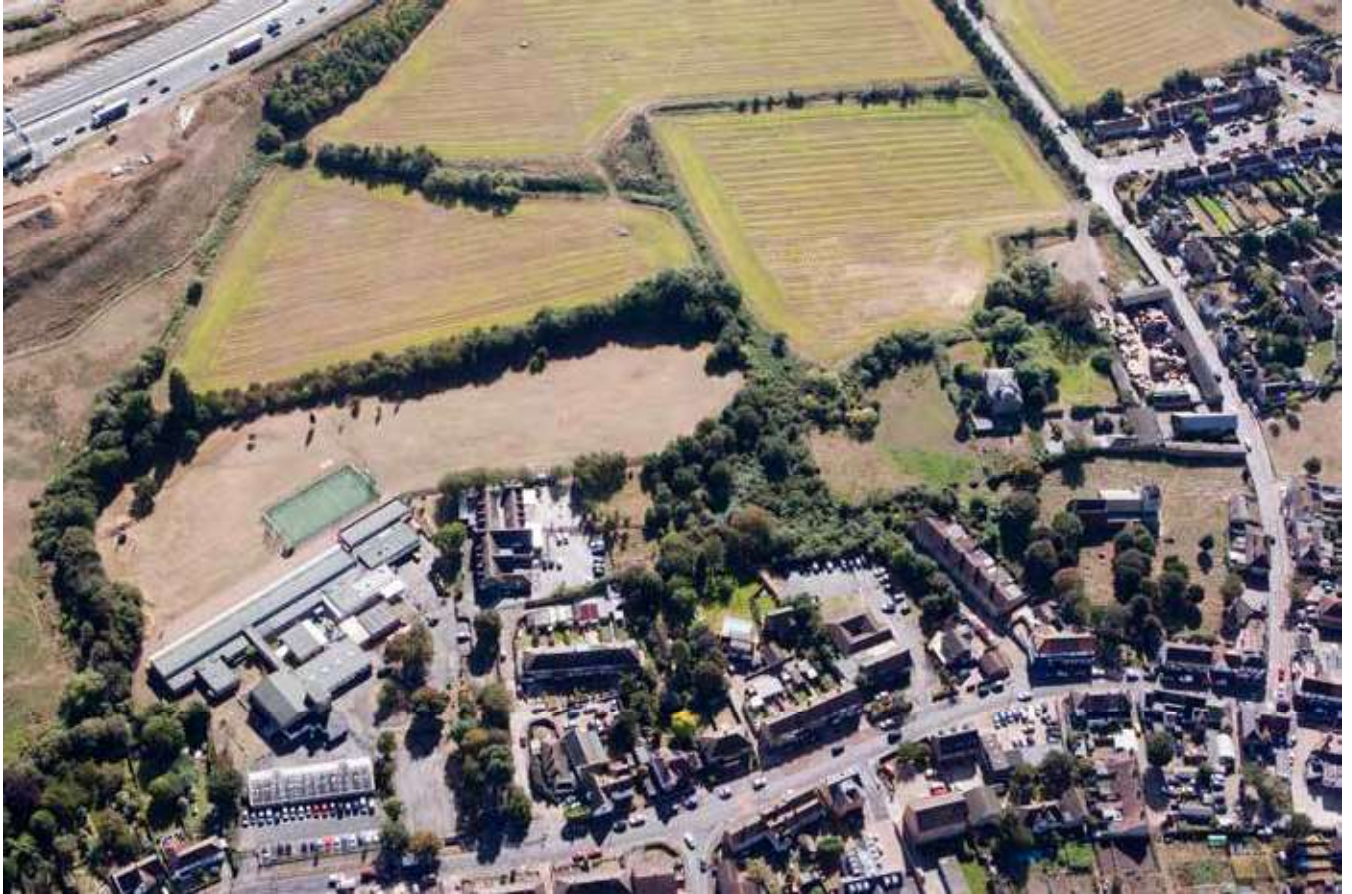
Figure 28: Aerial photograph of the Scheduled moat in the centre, with the church of St Michael and post-medieval Aveley Hall to the right and the A13 in the top left-hand corner.
