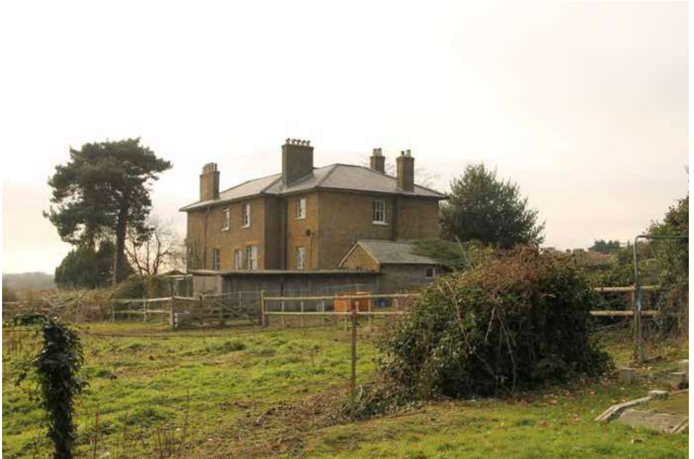
View 3: Looking from the corner of the moated site to Aveley Hall
