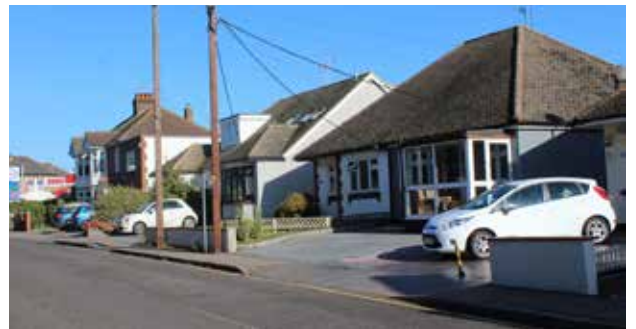
Figure 48: East side of Church Road
