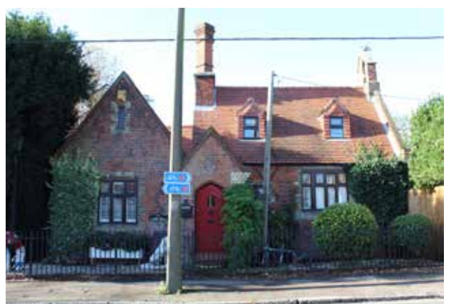
Figure 52: The Former School House
