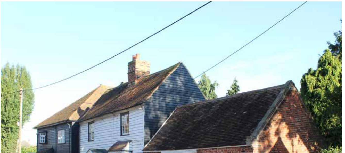
Figure 58-60 (clockwise from top left): Examples of roofing
