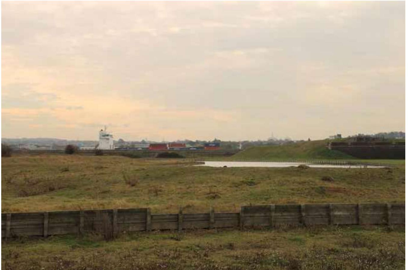
View 5. View from the landward side of Tilbury Fort to the river, the top of a cargo-ship is visible over the sea-wall, with Kent beyond it.
