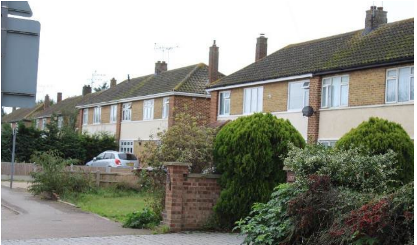
Figure 65: Boundary treatment and garden planting
