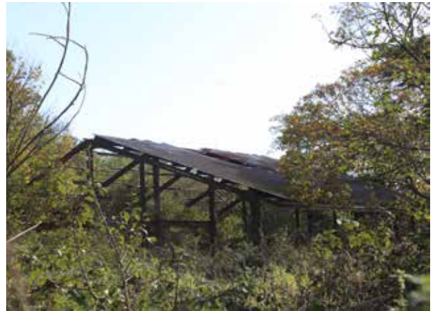
Figure 50: Structure remaining in the former Rectory grounds
